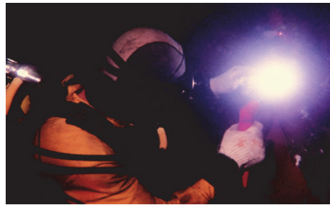
Fig. 2. Underwater welding with SMAW.
