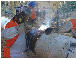
Fig. 30. Pipeline manual welding procedure.
